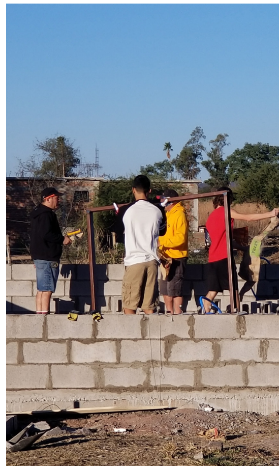
▼ Working at the construction site
